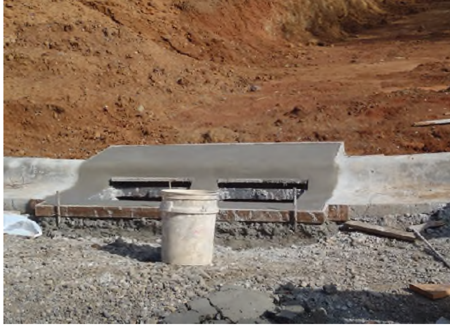
Figure 10 – Photograph showing collector boxes installed
